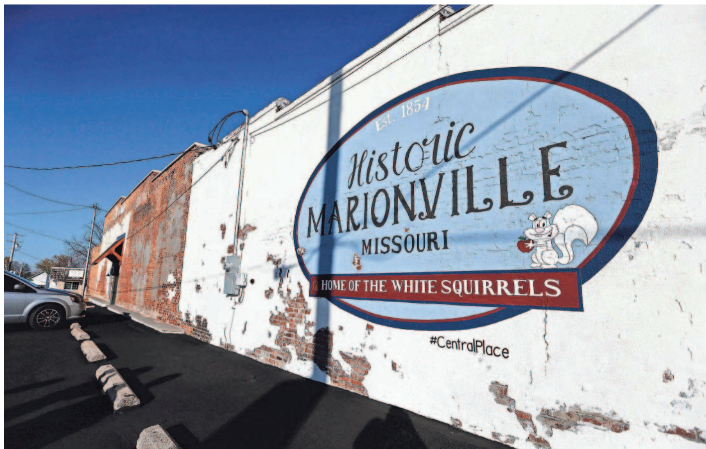
A mural on the outside of the building in downtown Marionville that Jim and Martha Brangenberg bought and renovated. The couple hope to bring “flourishment” to Marionville with the renovation of the 150-year-old downtown building.
